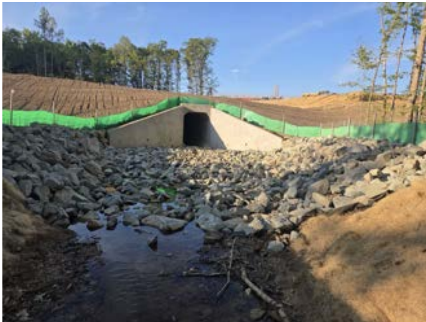
Image 14: Ponding on South side of the new access road. Measurement point for S1-4 was covered by the concrete and is near the center of the concrete box covert. Photo taken June 21st.
