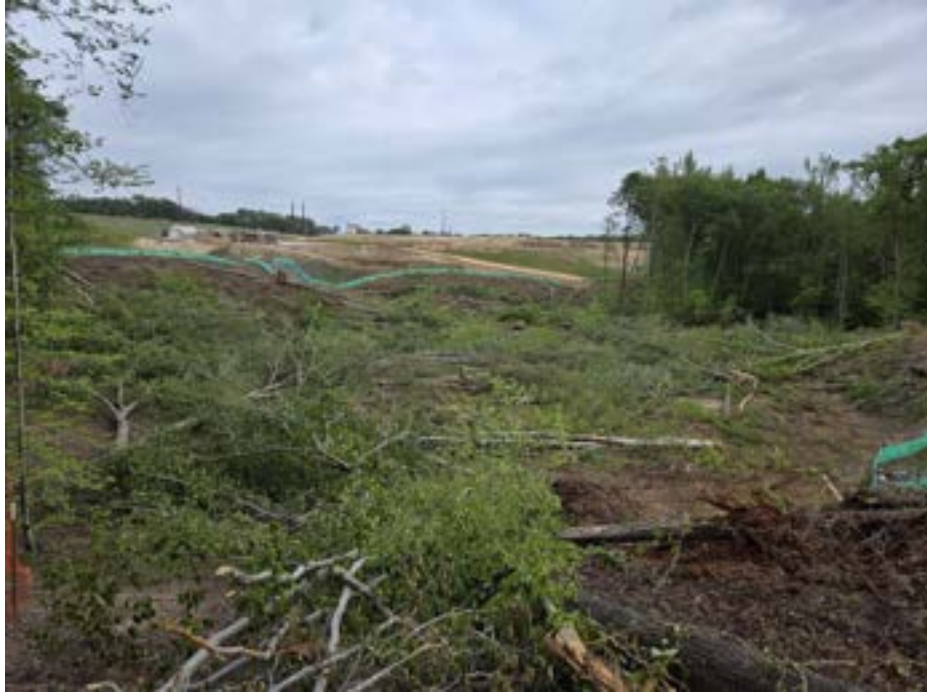
Image 7: Approximately 400 feet of trees were clearcut and left inside of Stream 1 for a new road that will connect to Eskimo Hill Road. Photo taken April 26th.
