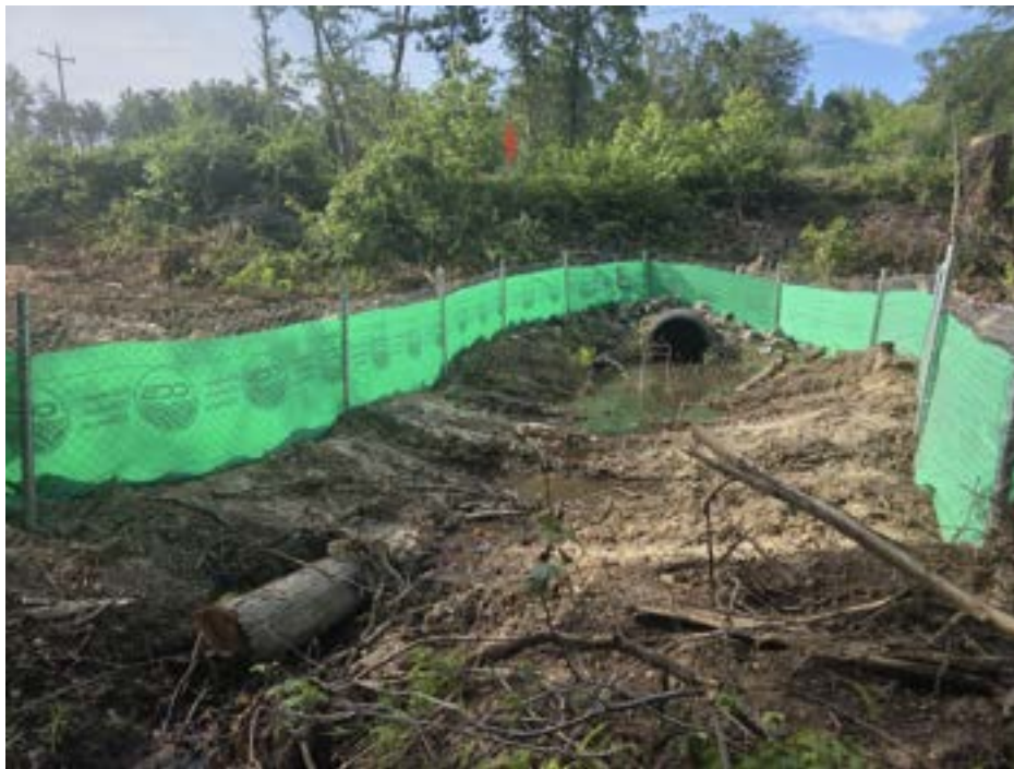
Image 6: Slash left in Stream 3 south of Eskimo Hill Road and deep tire tracks create an uneven path for water. Photo taken June 21st.
