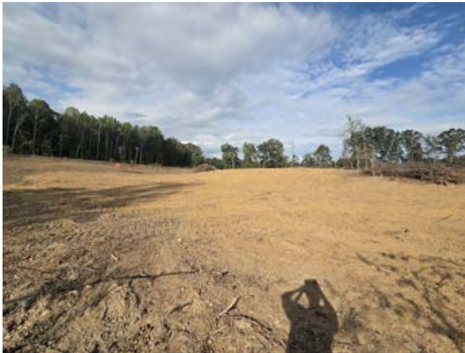
Image 4: Trees removed south of Eskimo Hill Road. The entirety of Eskimo Hill Road going through the STC site is similar in appearance. Photo taken June 10th.
