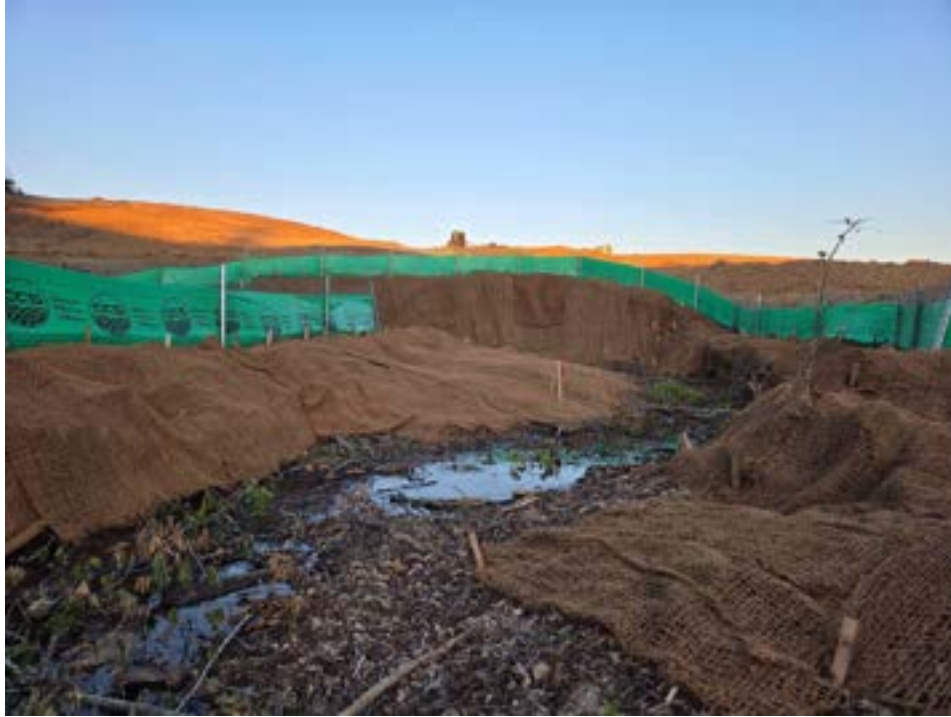
Image 9: After clearcutting and trees were removed from the stream. Photo taken in the same location shown above on May 3rd.
