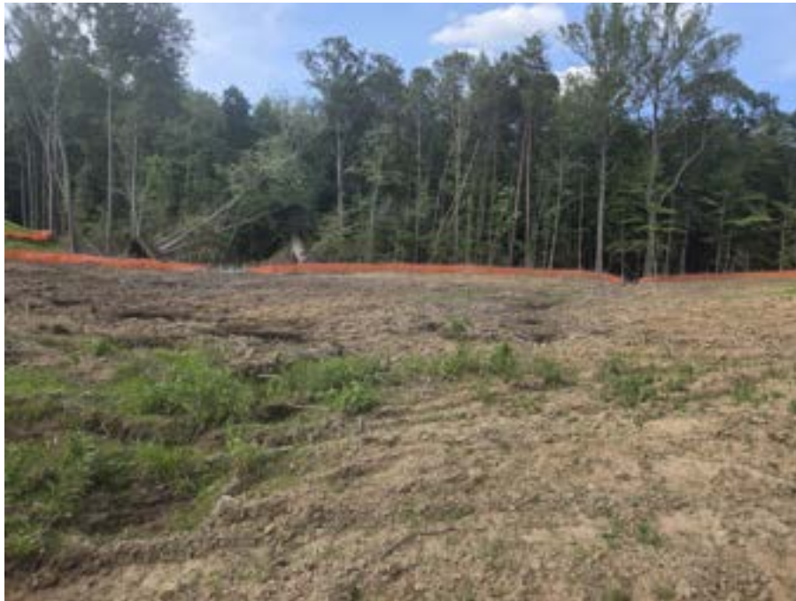
Image 21: Previously forested land was graded along Eskimo Hill Road. Measurement point for S3-1 is where the orange barrier is not present on the left. Photo taken June 21st.
